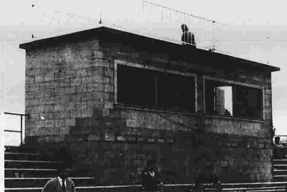
New press box stands at Manchester High School's Memorial Field, replacing the old one, which had been condemned by officials. The new facility is roomier than the one it replaces and also has storage area underneath for athletic equipment. It was constructed by school personnel.
